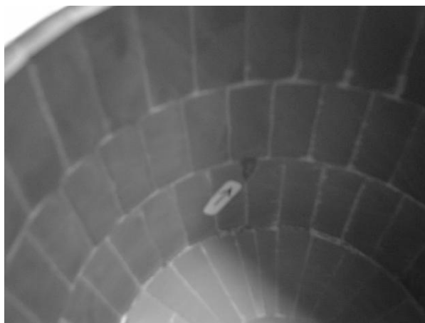
Figure 13: one of two cracks in the lining plates, both appeared in cylinder-lining
