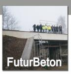
the world's first public bridge made of High Performance Cement/Concrete
